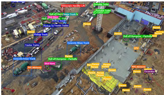
SITE INTELLIGENCE Offsite processing or even in-camera AI analysis can tag equipment, workers, materials and identify unsafe conditions.
